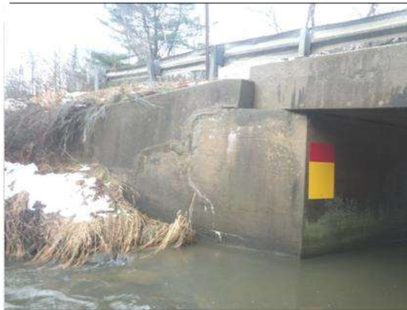
Down stream West wing wall
