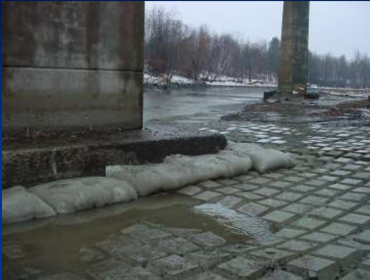
Articulate concrete block mat
