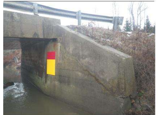
Down stream East wing wall
