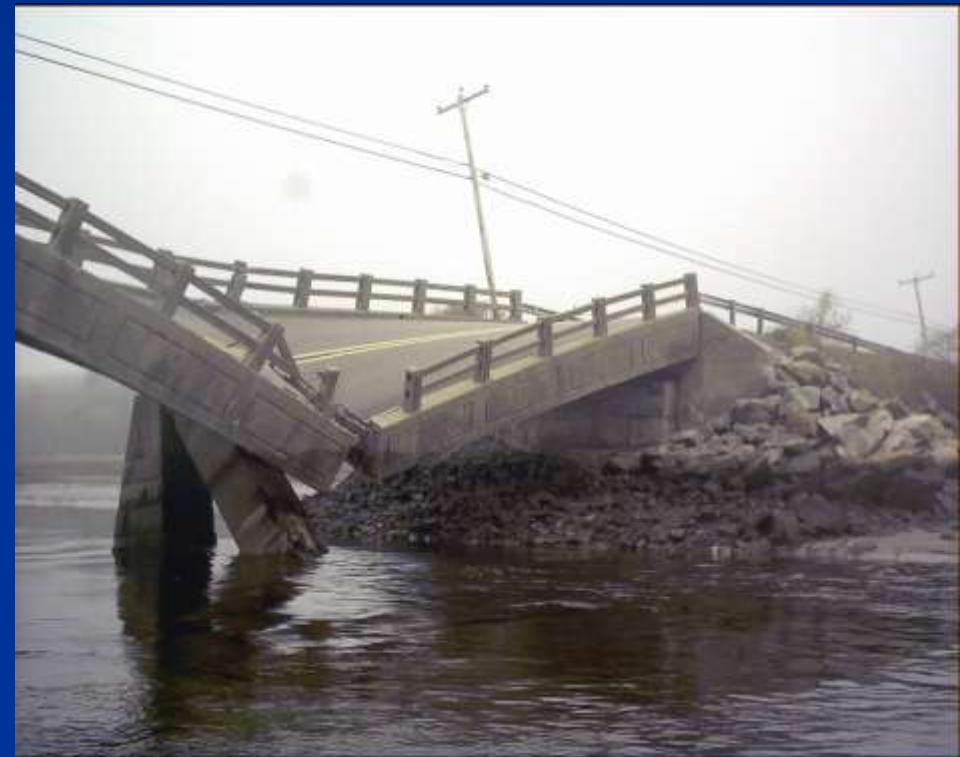
AFTER FLOOD (15 inches of rain in 36 hours)
