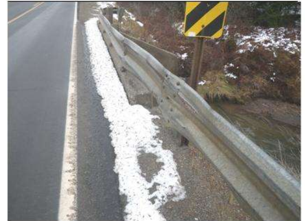
Typical collision damage to approach and bridge rail.
