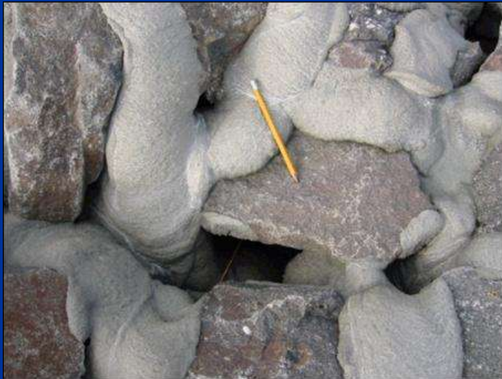
Partially Grouted Riprap
